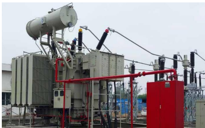
Power Transformer supplied for Bhopal Metro Project
