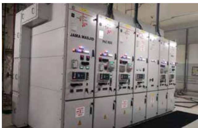
GIS Supplied for Underground Substation (Agra Metro Project)
